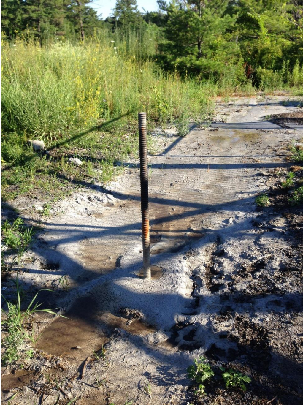
Figure 4-2. Sacrificial hollow bar micropile prior to load testing
