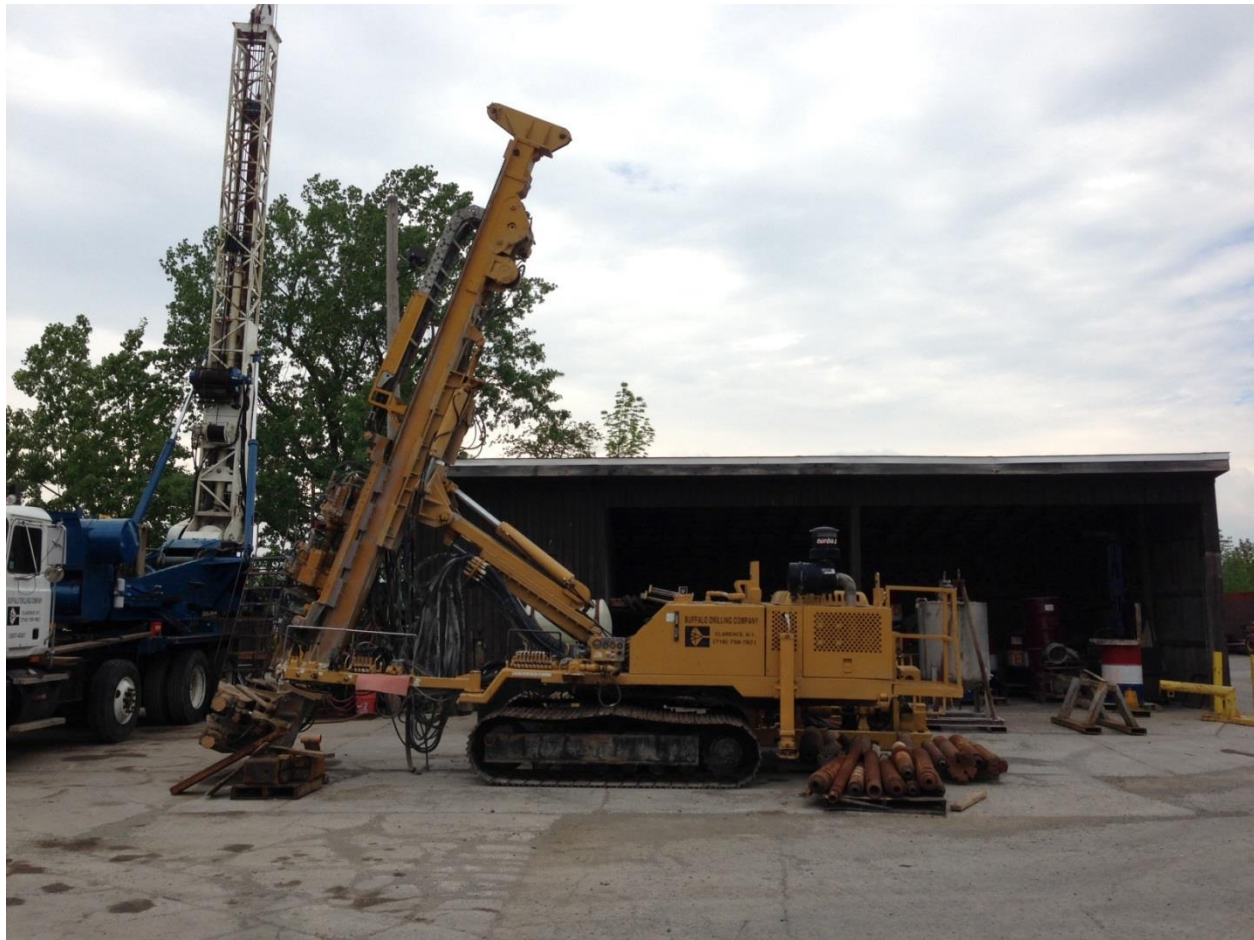
Figure 3-2. Davey Kent 725 drill rig used for micropile construction
