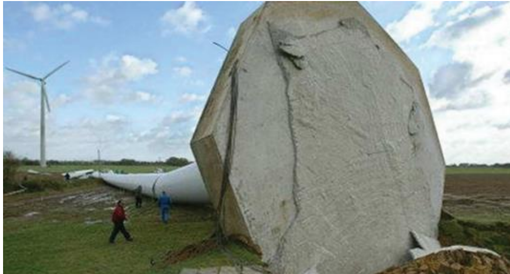
Figure 1-11. Overturned shallow foundation of a wind turbine (Aschenbroich)
