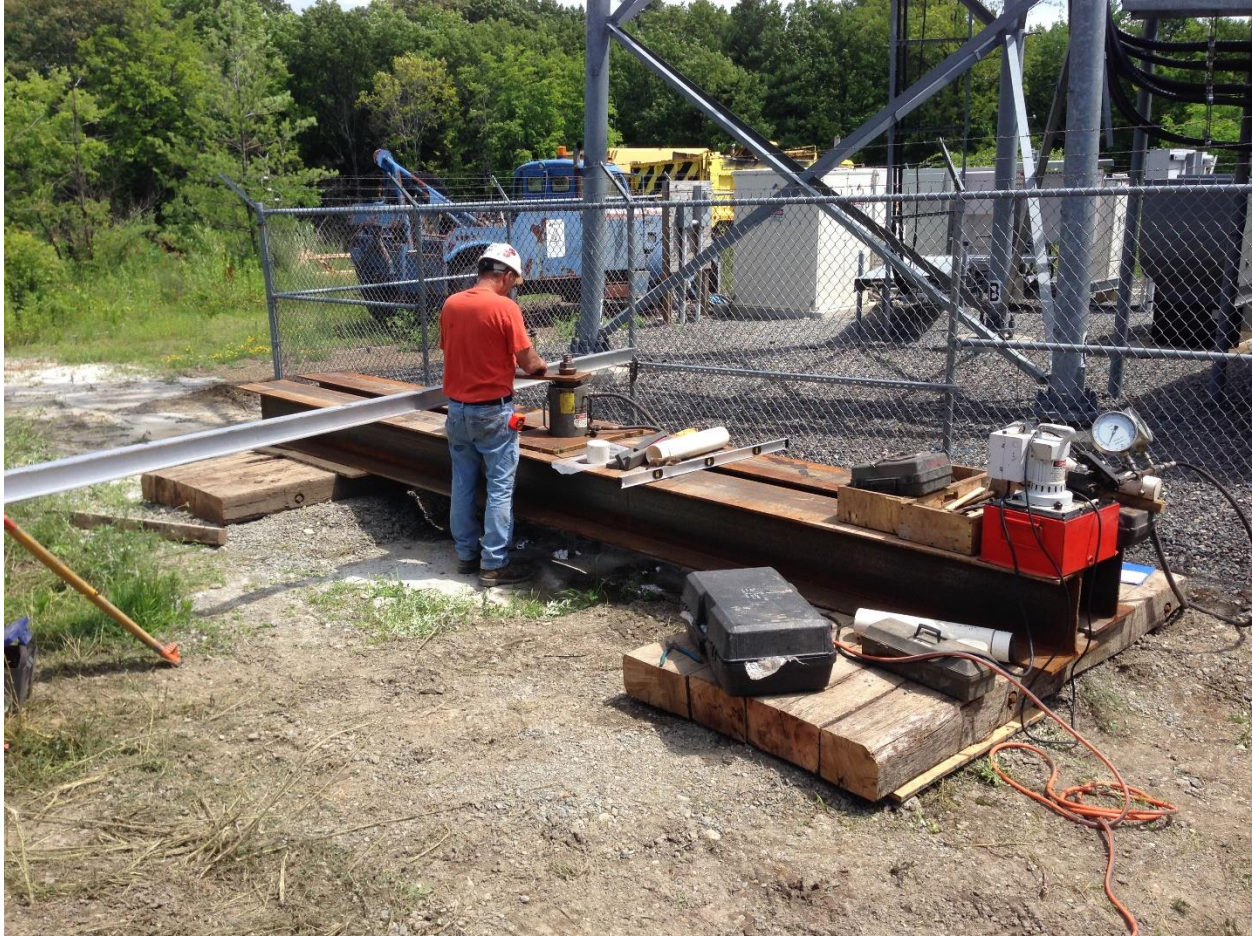
Figure 4-1. Micropile static load test setup prior to applying tensile load
