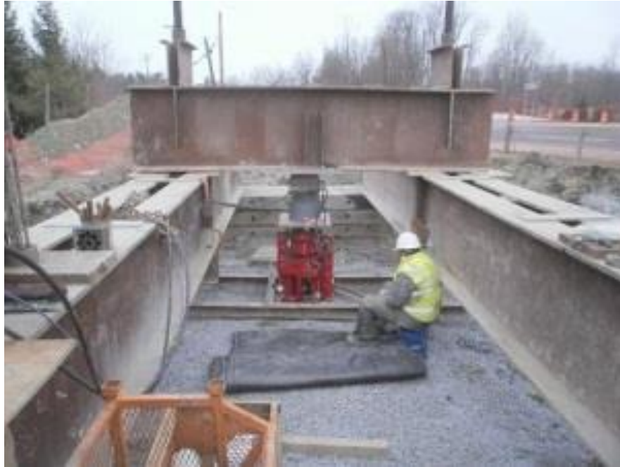
Figure 6-6. Micropile load test setup
