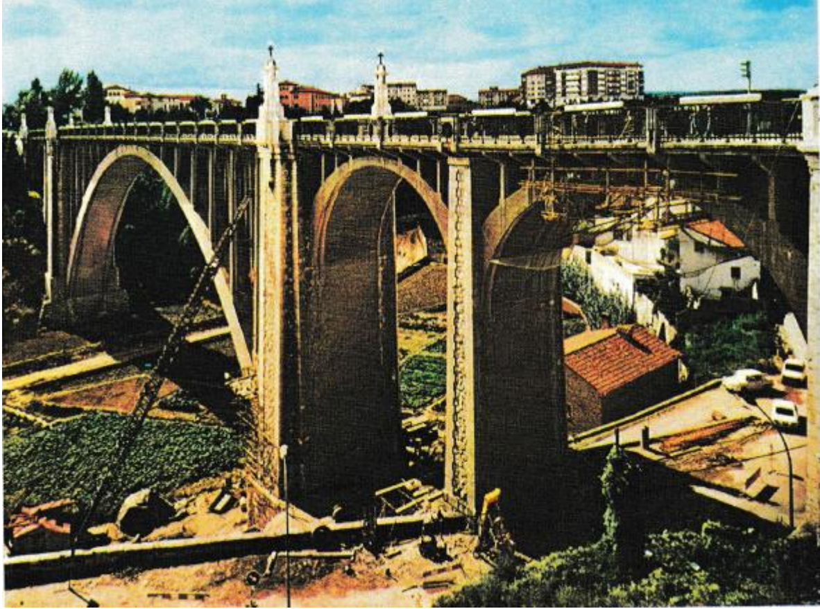
Figure 1-17. Viaduct pali radice construction done in Teruel, Spain (Lizzi, 1982)
